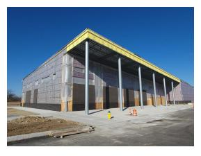
Progress continues on the 16 acre project as our General Contractor, Brumbaugh Construction has the building nearly "buttoned up" for winter. Most all of the sidewalks and curbs have been poured, insulation is on the building, exterior brick work is complete and temporary plastic has been installed to all future window openings.
